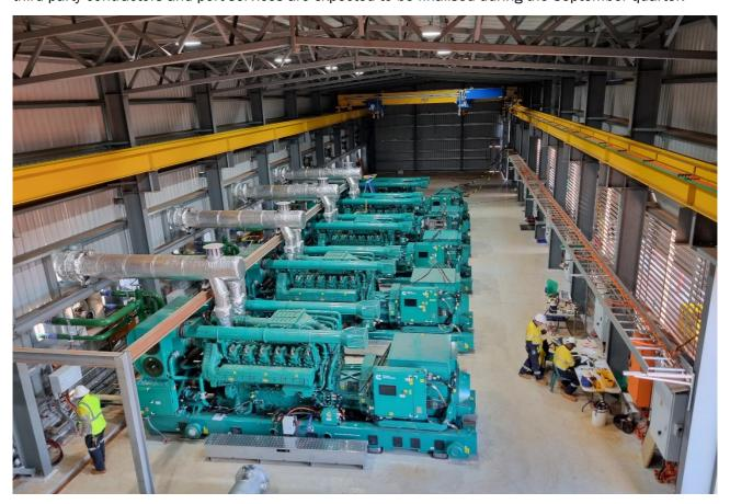
Figure 5: Progressive installation of power generation units underway
