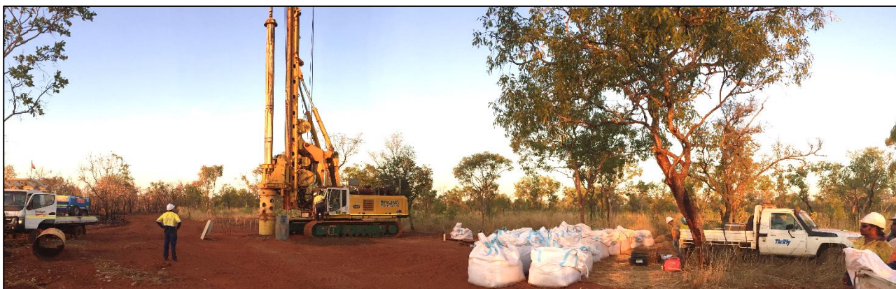
Figure 4: Bulk sample collection with a Bauer rig
