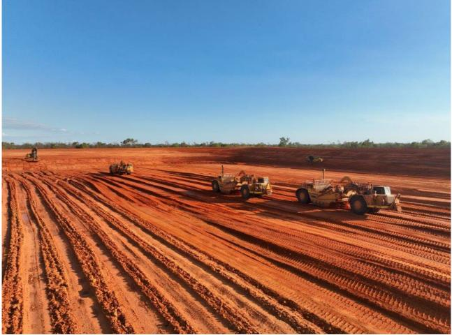
Image 5 & 6: Tailing storage facility construction & contouring activities
