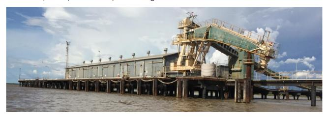
Figure 2: Derby wharf with bulk export ship loading facility
