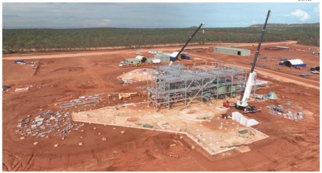
Image 1 & 2: Thunderbird Plant Site Progress – Plant steel erection and process tank installation
