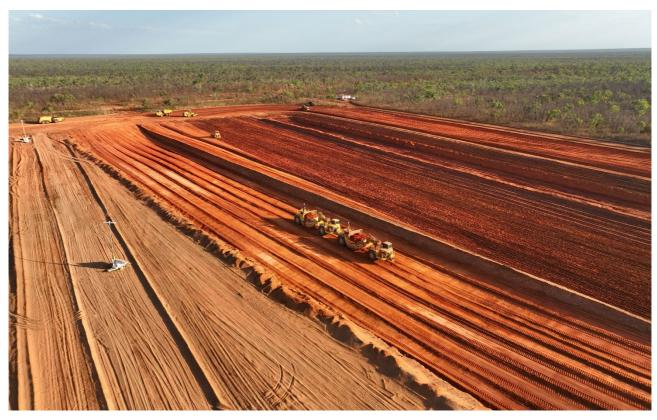
Figure 3: Construction of Tailings Storage Facility underway at Thunderbird
