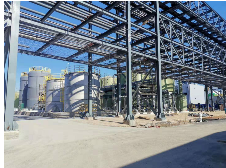
Tank Farm Source: Yansteel
