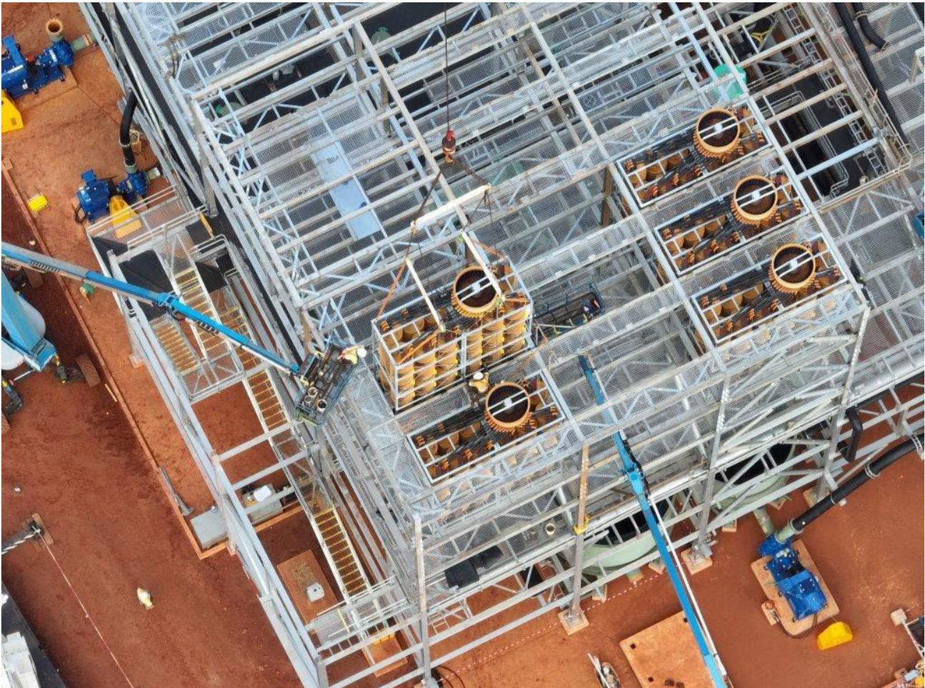
**Figure 7: Installation of spirals underway**
