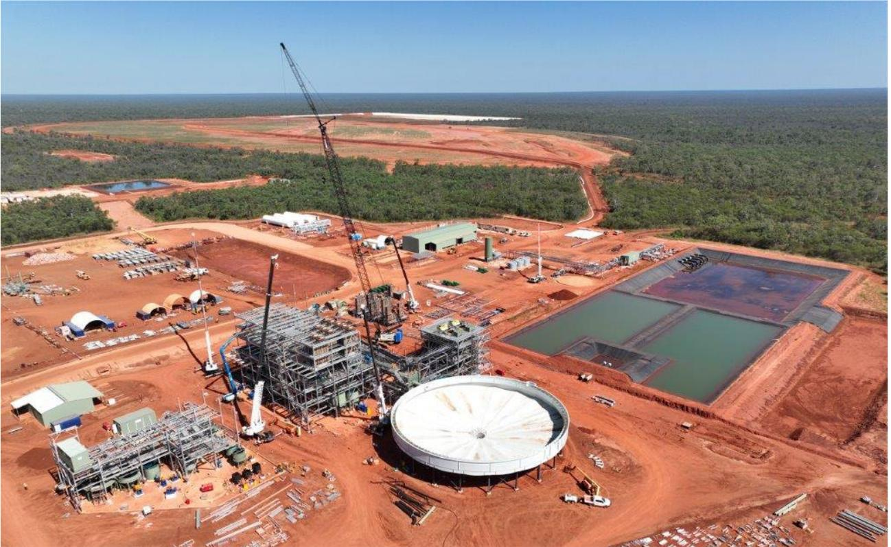
**Figure 3: Thickener construction (foreground) with WCP construction in progress**
