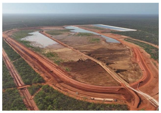
Figure 6: Tailing storage facility, with planned wall lift (foreground) underway
