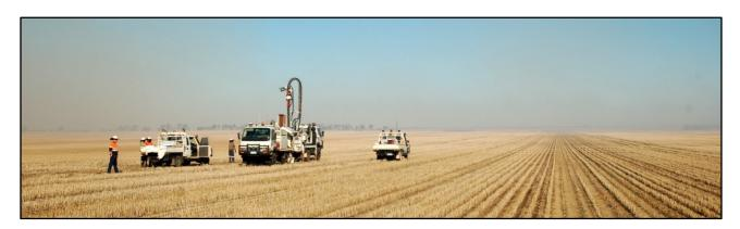
Figure 12: Aircore drilling at the Yandanooka Deposit
