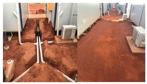
Figure 5: Completed mine accommodation stormwater piping & contouring
