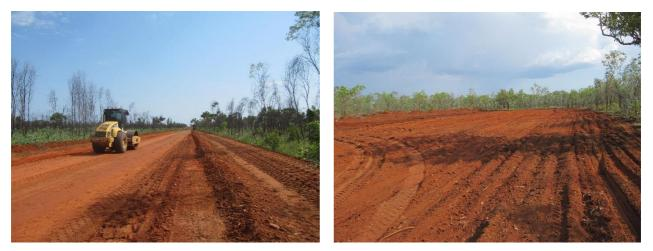
Figure 2 & 3: Site access and clearance of accommodation area underway at Thunderbird
