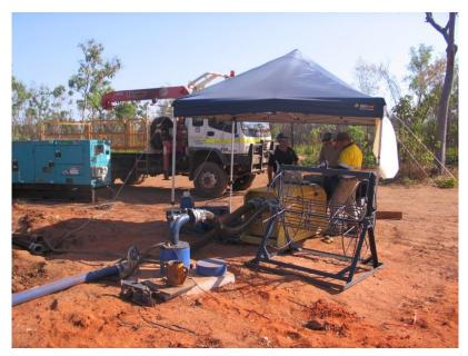
Figure 7: Groundwater pump testing at Thunderbird
