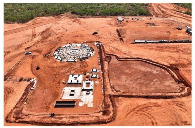
Figure 2: Process Plant area – Initial concrete installation
