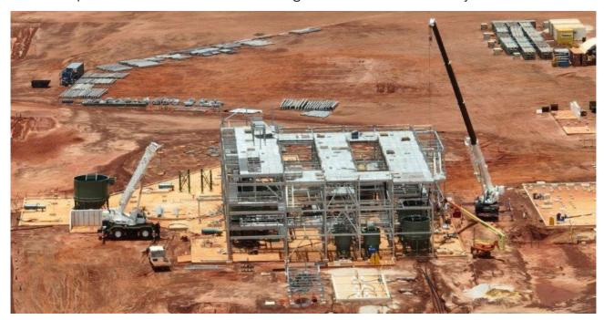
Figure 2: Wet Concentrator Plant steel installation
