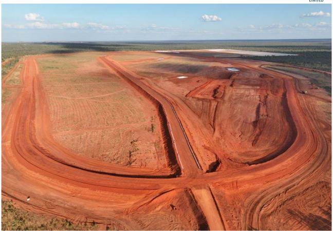
Image 7: Tailings storage facility (foreground) and stormwater storage pond (background)
