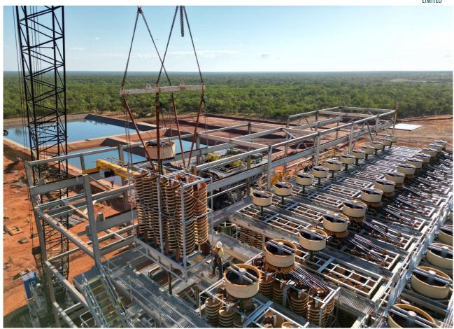
Image 3 & 4: Final set of spirals installed at Wet Concentrator Plant
