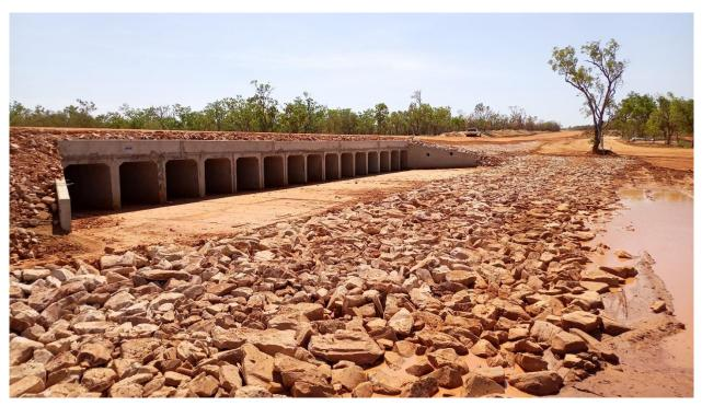
Figure 3: Thunderbird mine access road – culvert installation
