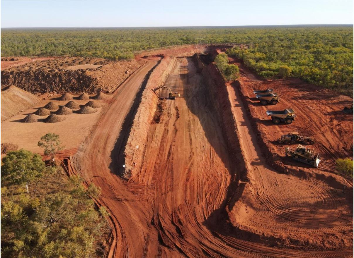
**Figure 3: Mine trial pits 1 & 2 and ore and waste stockpiles**
