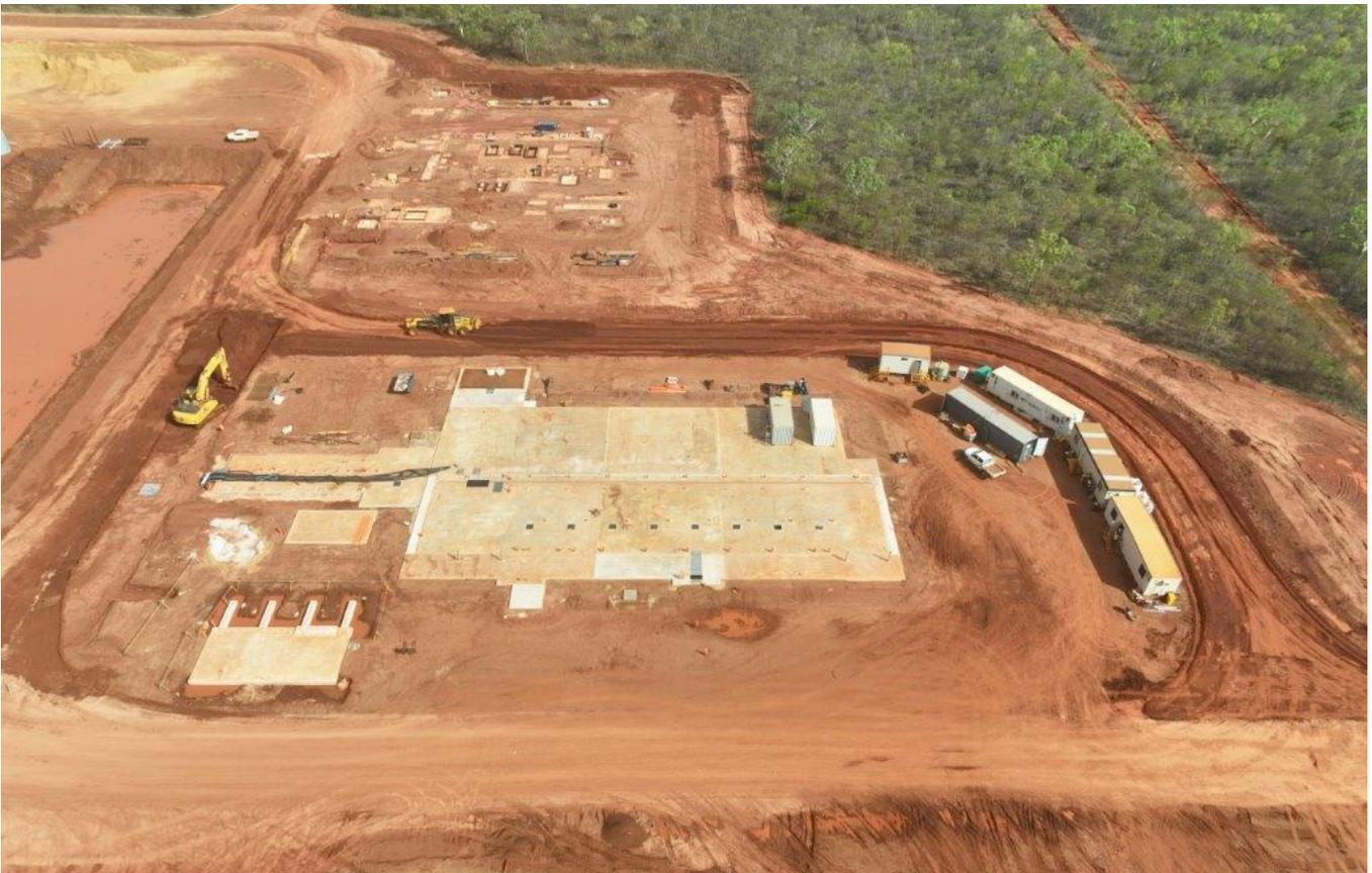
Image 4: Power Station concrete works completed ahead of installation by Pacific Energy Pty Limited
