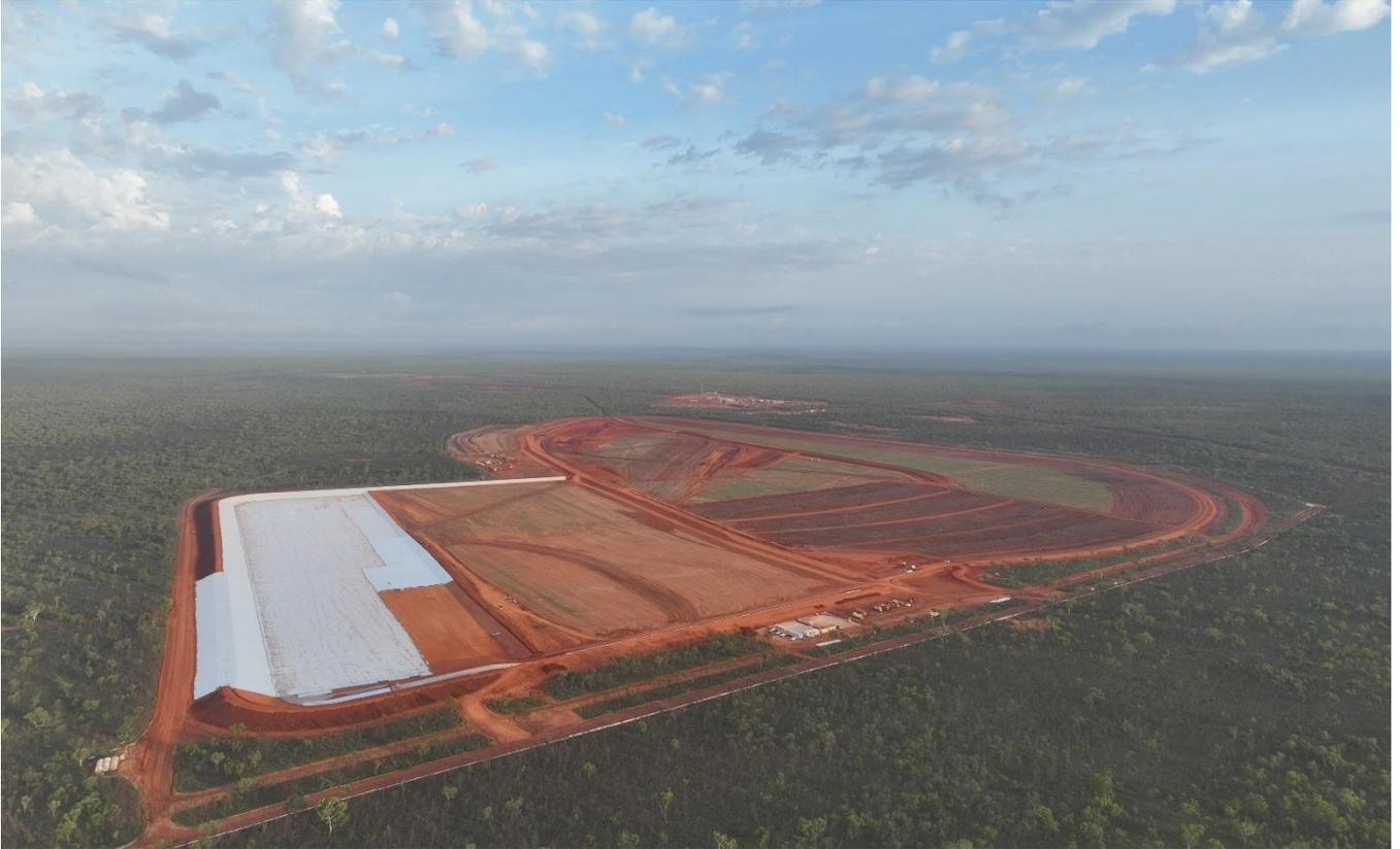
Image 3: Lining of the Stormwater Storage Pond underway
