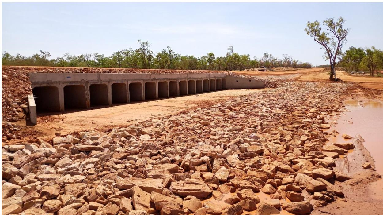
Figure 2: Thunderbird mine access road – culvert installation
