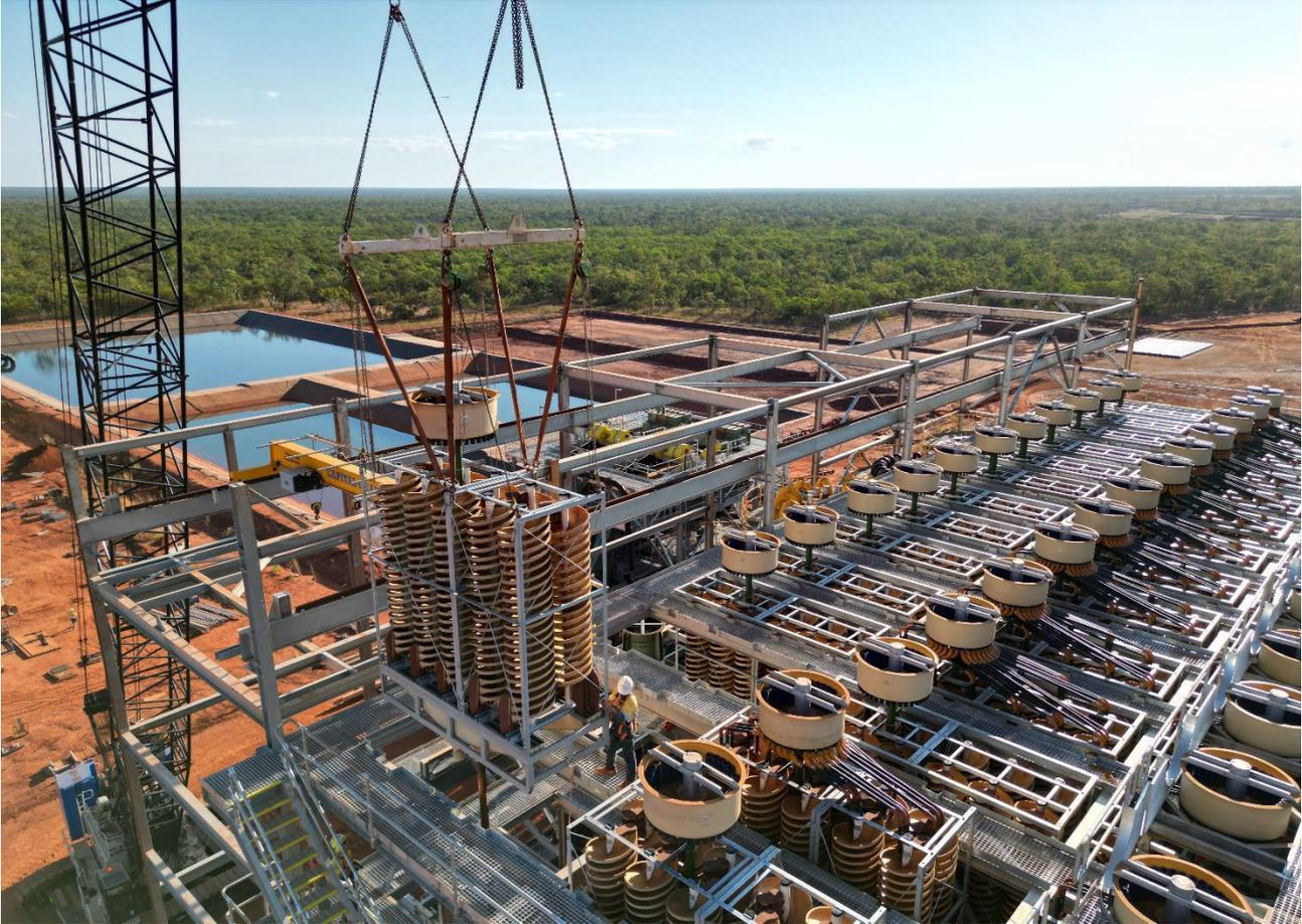
Image 3 & 4: Final set of spirals installed at Wet Concentrator Plant
