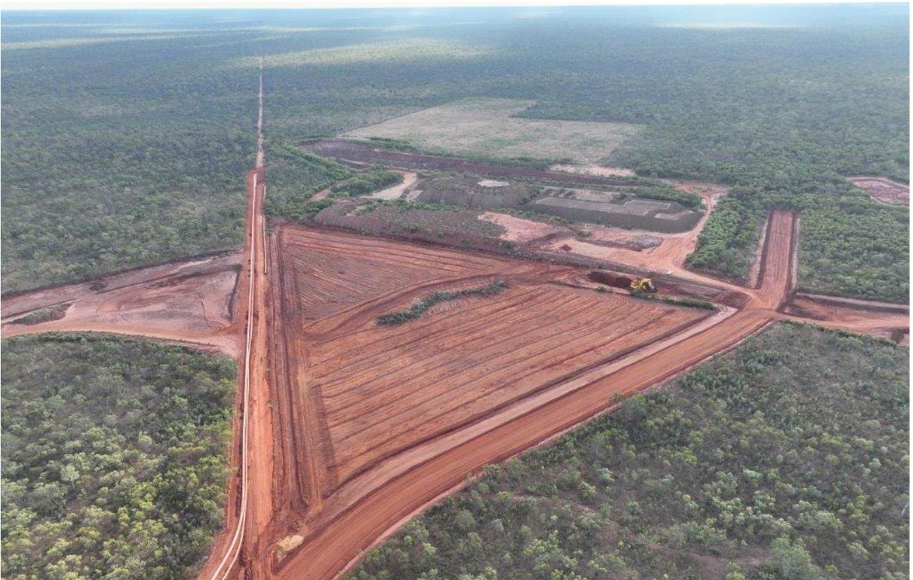
Image 8: Commencement of clearing & grubbing for overburden stockpile area
