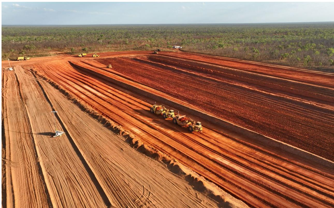
**Figure 3: Construction of Tailings Storage Facility underway at Thunderbird**
