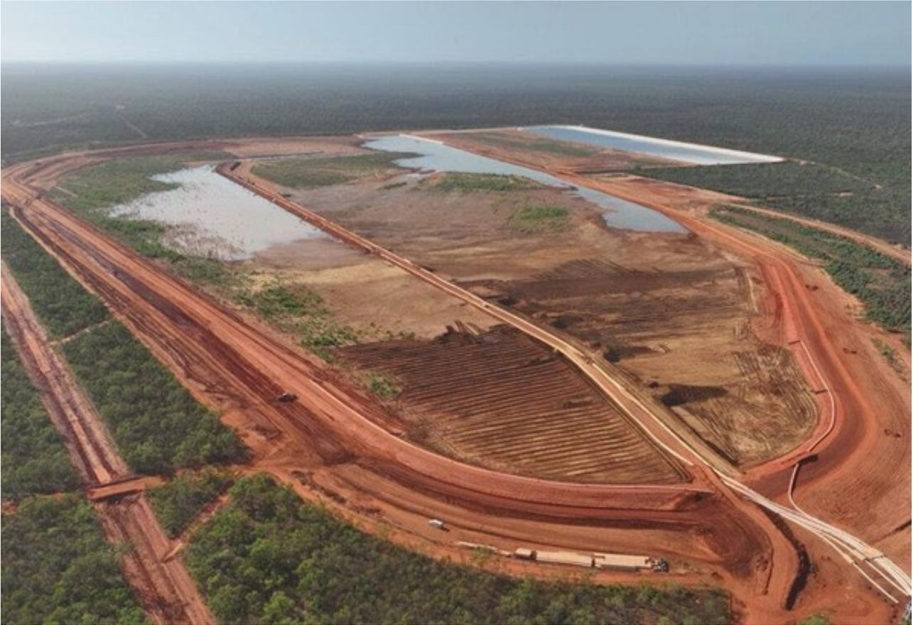
**Figure 6: Tailing storage facility, with planned wall lift (foreground) underway**
