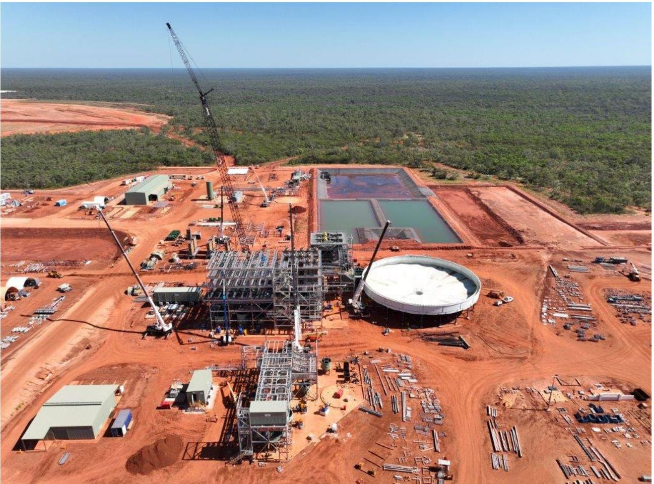
**Figure 4: Concentrate Upgrade Plant (foreground) construction in progress**
