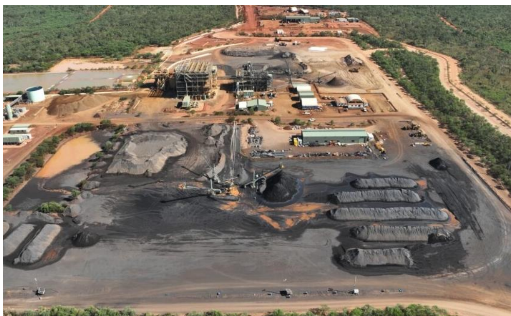
Figure 1: Thunderbird Process Plant & stockpile area
