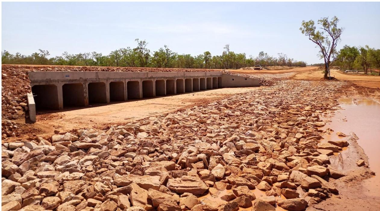
Figure 2: Thunderbird mine access road – culvert installation
