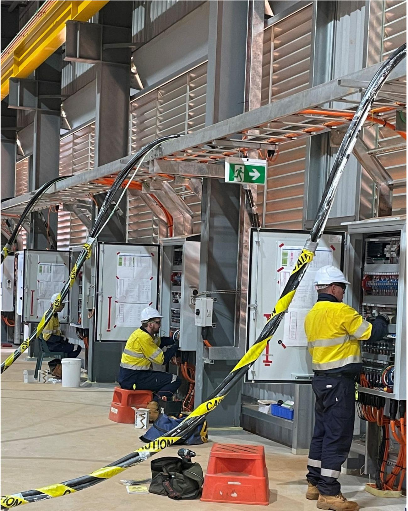
Image 8: Power station switchboard installation underway
