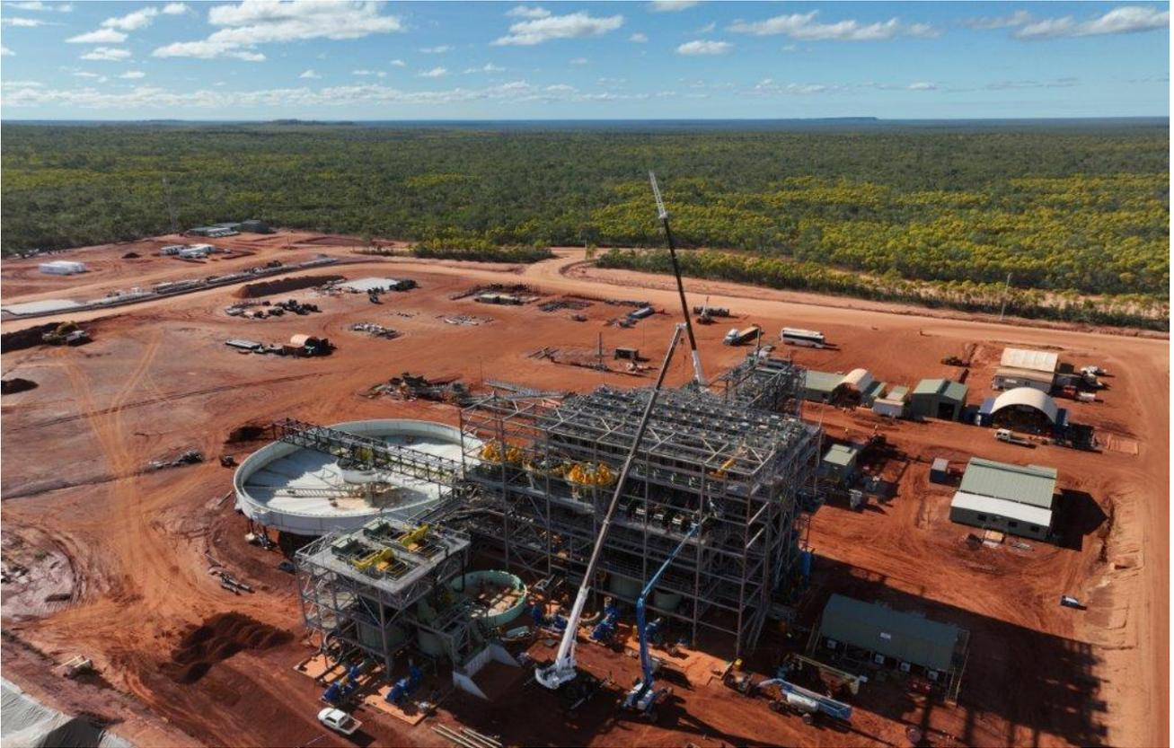
**Figure 3: Wet Concentrator Plant construction in progress**
