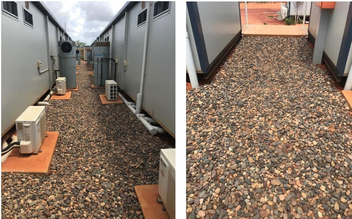
**Figure 1: Completed River Gravel between Accommodation units**
