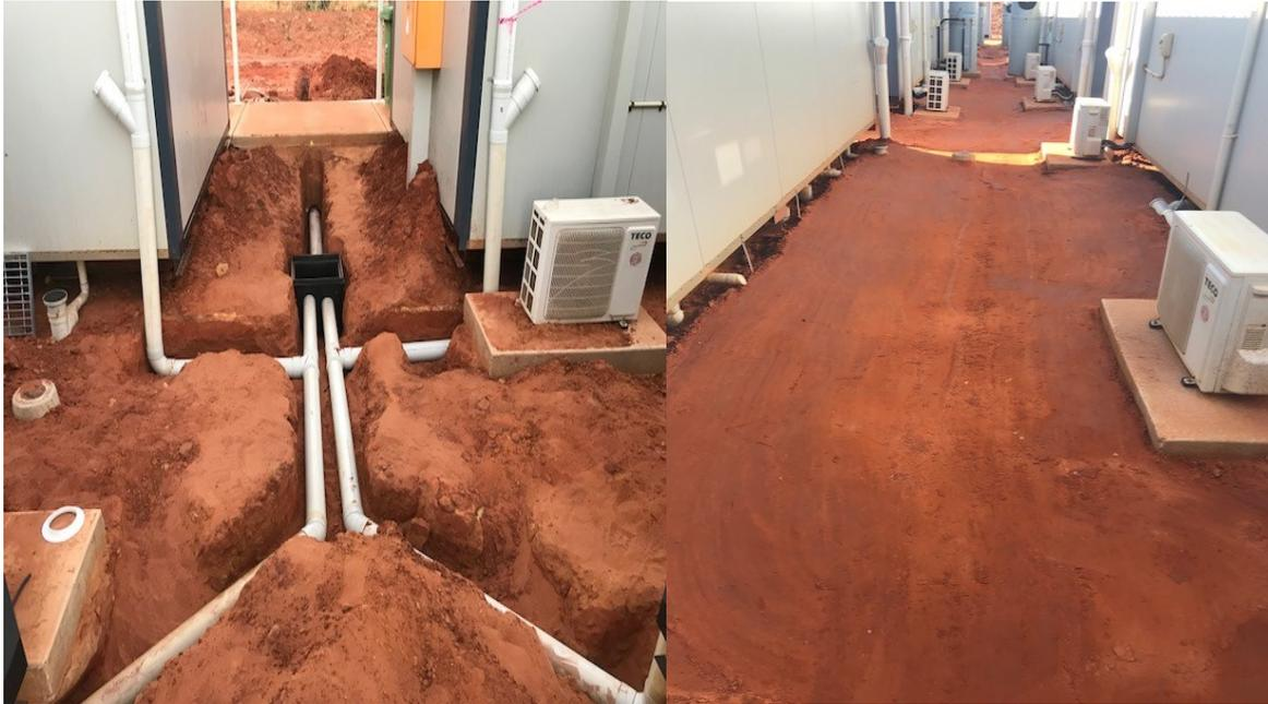
**Figure 5: Completed mine accommodation stormwater piping & contouring**
