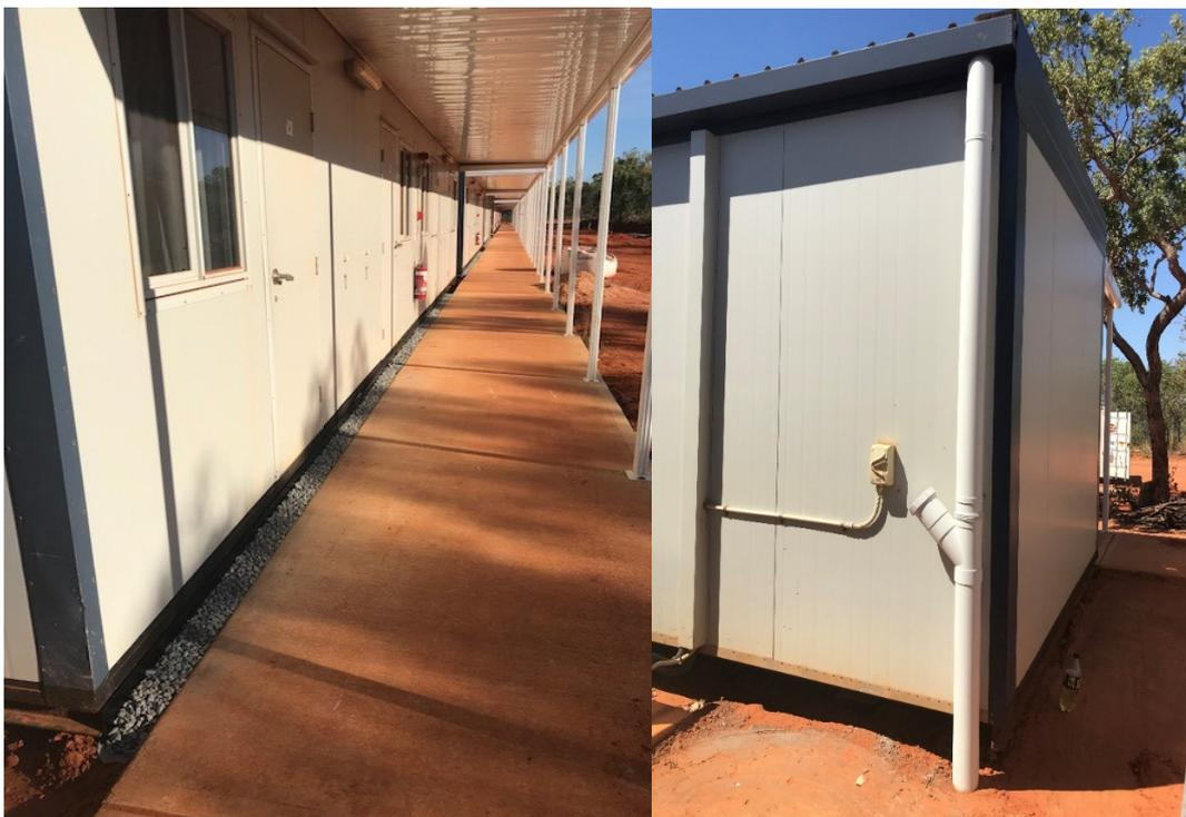
**Figure 6: Mine accommodation flat bar and blue metal installation & painting of PVC piping**
