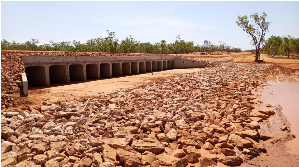
Figure 3: Thunderbird mine access road – culvert installation
