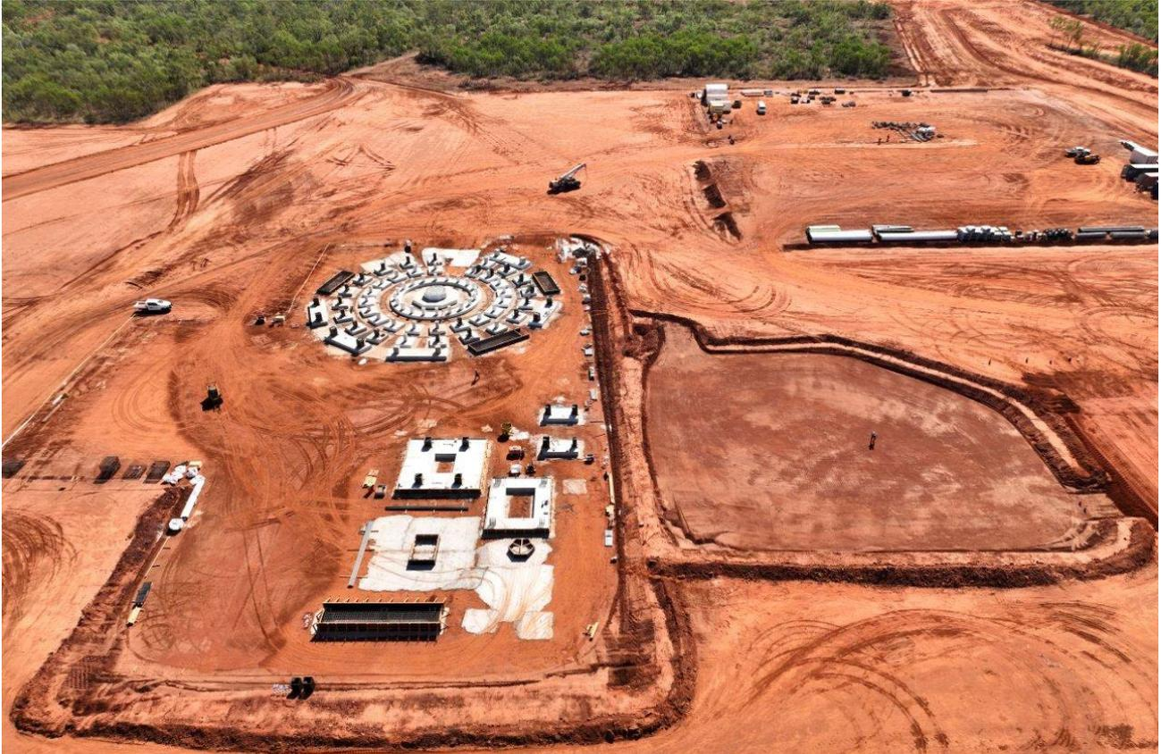
Figure 2: Process Plant area – Initial concrete installation
