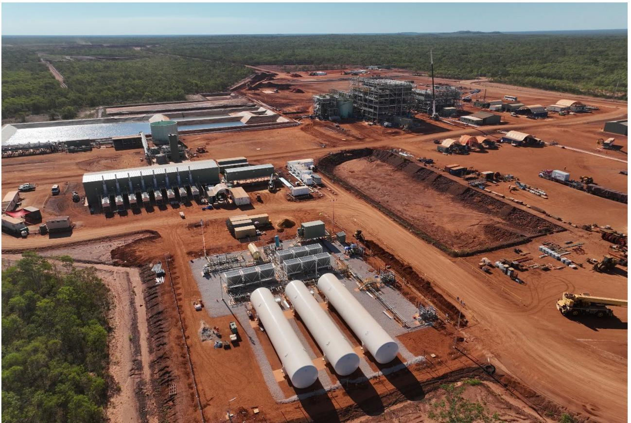
Image 4: Overview of Power Station & LNG Storage Tanks (foreground)
