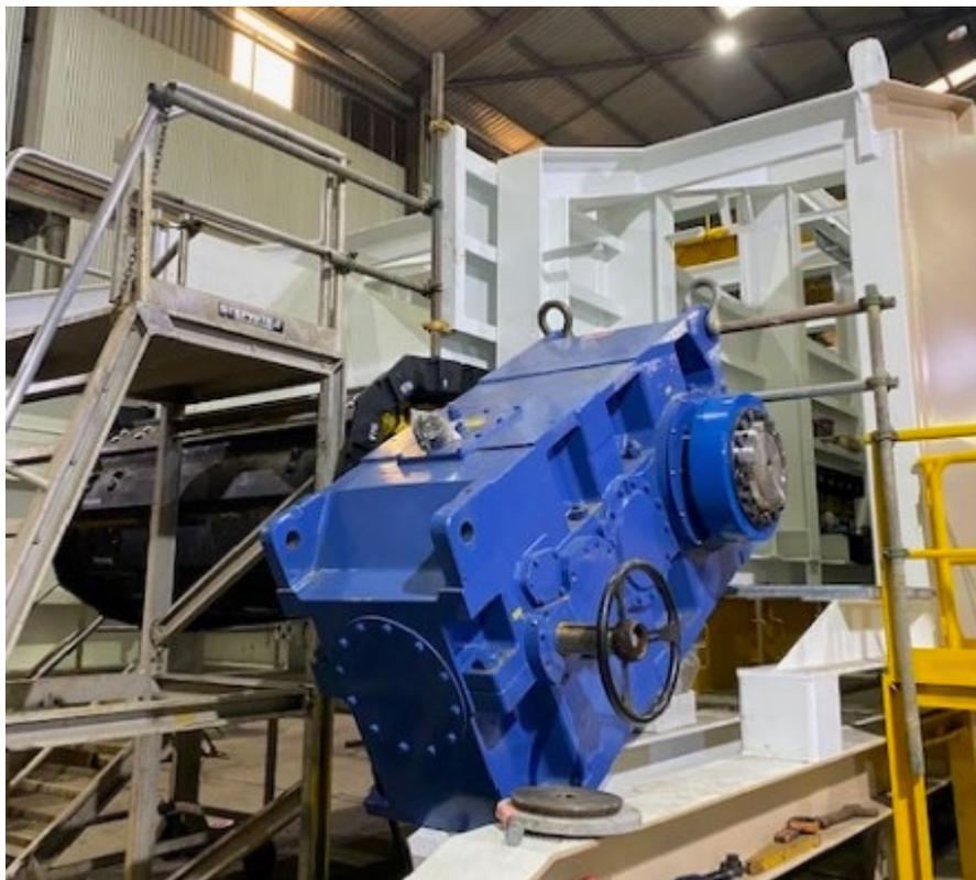
Image 6: Installation of Dry Mining Unit Drive Assembly
