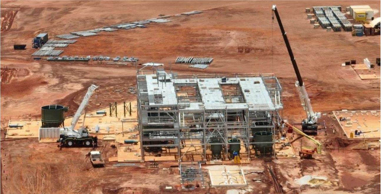
Figure 2: Wet Concentrator Plant steel installation
